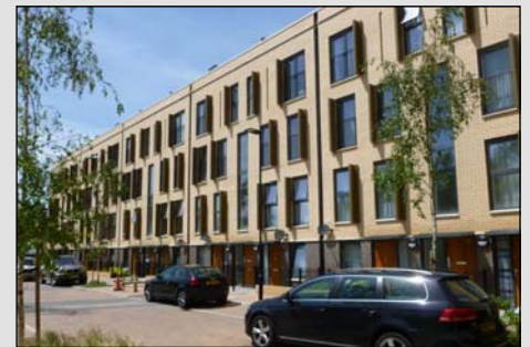
View of the completed 4-storey residential accommodation
