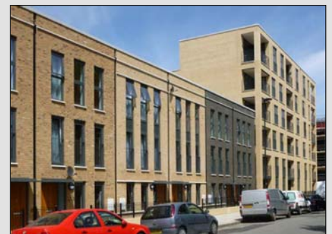
Featured brickwork supported by the light steel structure
