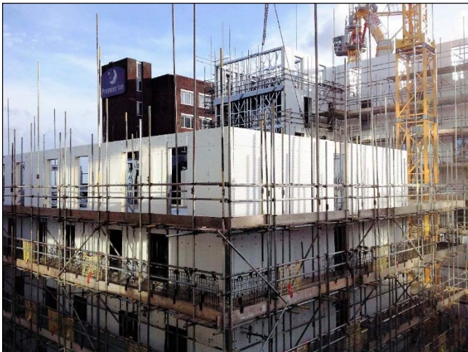
Installation of light steel framing with pre-clad external walls
