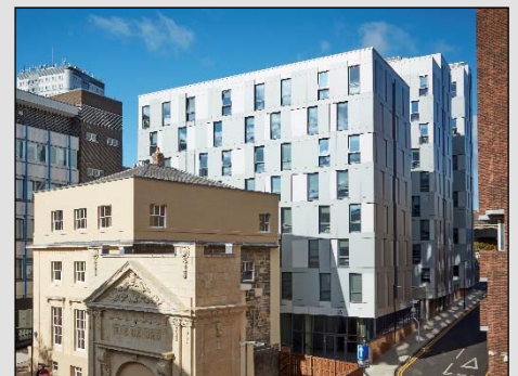
Completed 10 and 12 storey blocks
