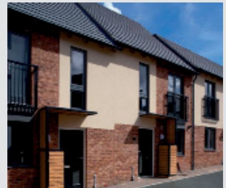
Light steel frame housing development in Leeds
