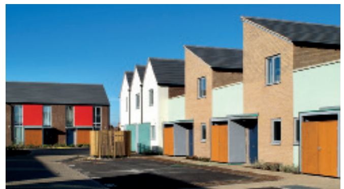
Figure 4 Light steel framing in Cambridgeshire studied in BRE SmartLIFE project
