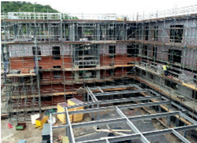
Figure 1 Construction of multi-storey light steel frame residential development
