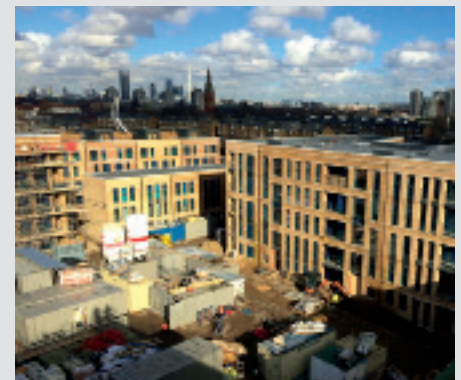
Large residential development using light steel framing in London
