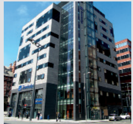
A 9 storey light steel frame hotel in Liverpool
