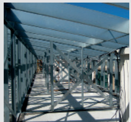
Load-bearing light steel walls with light steel roof joists
