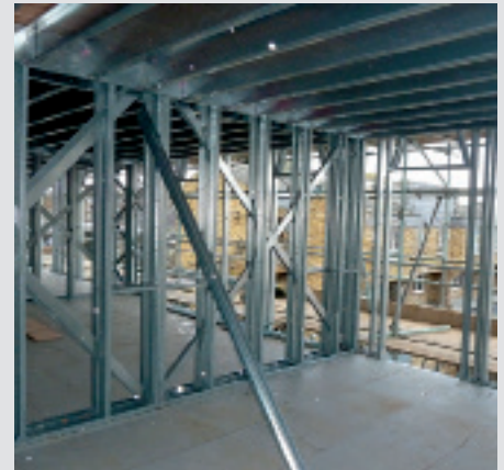
Wall panel supported by temporary struts
