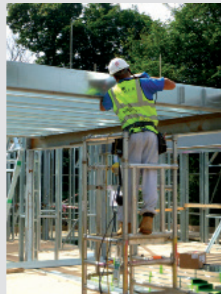
Floor joists installed from a moveable working platform
