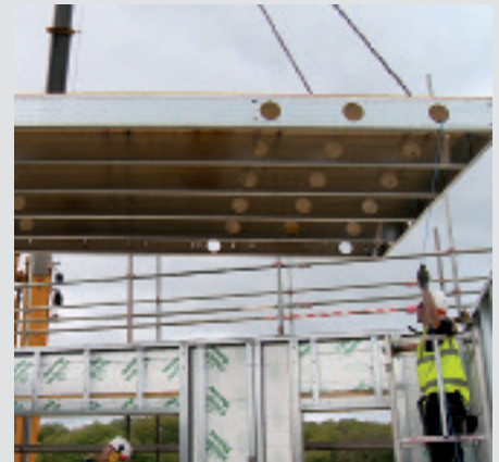
Installation of a light steel floor cassette
