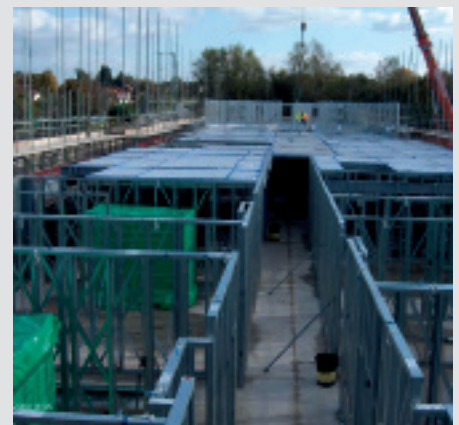
Wall panels installed with perimeter scaffolding
