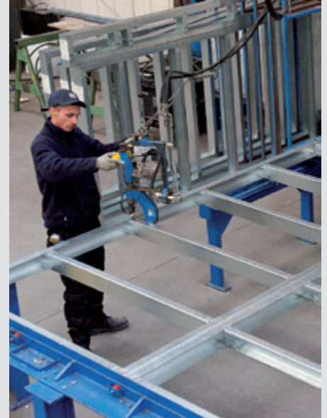
Manufacture of light steel wall panel within a factory environment after design freeze
