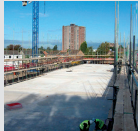
Ground floor slab with scaffolding installed around the perimeter
