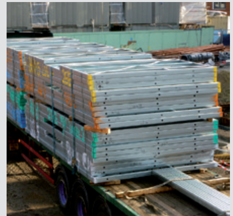
Delivery of wall panels on articulated vehicle with access to site
