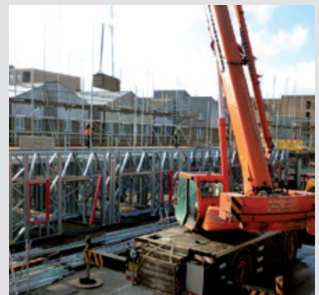
Crane lifting materials into position from agreed crane set area
