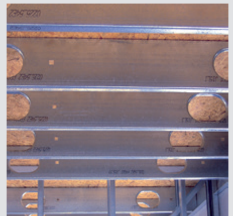
Light steel floor joists with large stiffened web openings
