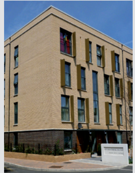
Brickwork external cladding on light steel frame building
