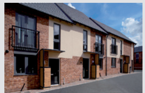
Two storey light steel housing (Image courtesy of Kingspan Profiles & Sections)
