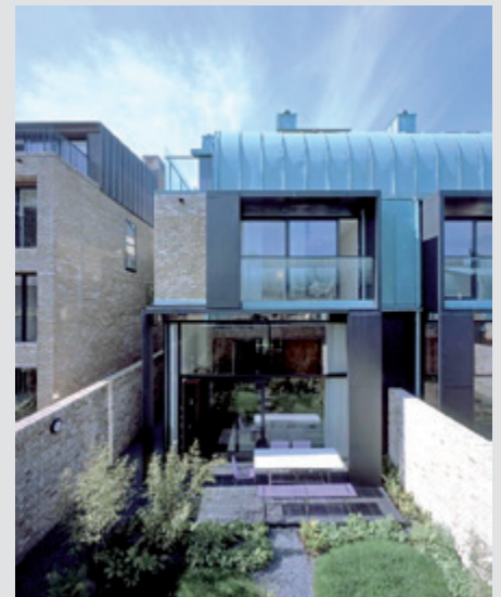
Town houses at Accordia, Cambridge (Image courtesy of Metek UK and Alison Brooks Associates)
