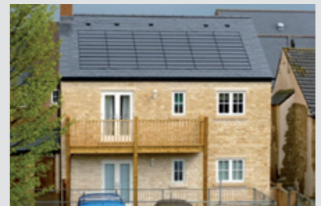
Code Level 5 houses at Bicester, Oxon (Image courtesy of Fusion Building Systems)
