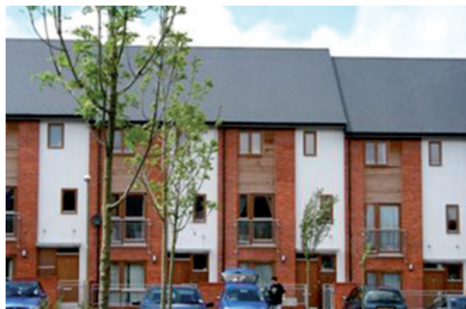
Figure 1 Three storey housing in Basingstoke (Image courtesy of Ayrshire Framing)
