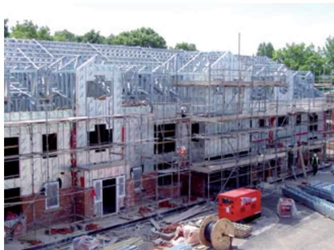
Figure 5 Light steel framing with open roof trusses in town housing (Image courtesy of Metek Building Systems)
