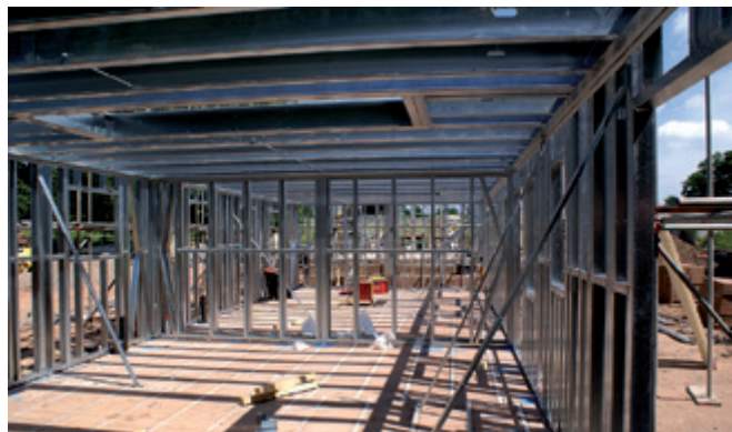
Figure 2 Light steel framing in housing (Image courtesy of BW Industries)
