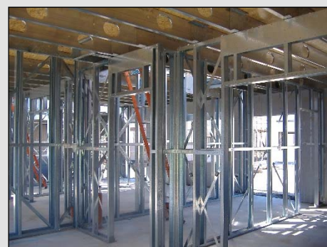
Fusion framing system during construction
