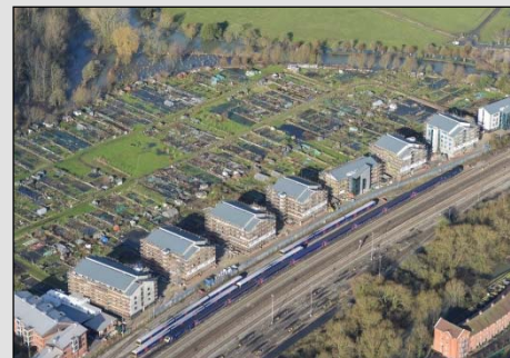
Aerial view of the completed project next to Oxford station
